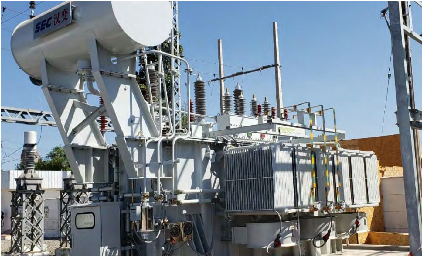
SFZ-30000 / 66 Power Transformer for LONGAVI Substation in Chile
